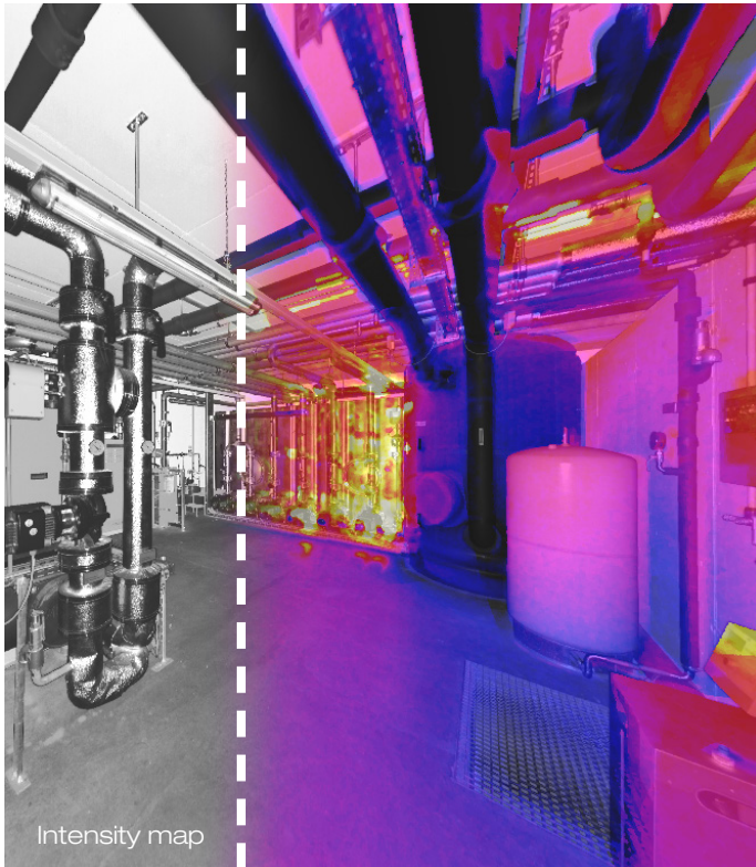
Point Cloud combined with thermal data
